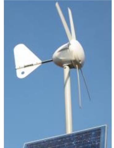
**Wiring from the turbine to the battery charger must be undertaken with the mast lowered and the windmill stationary.**
