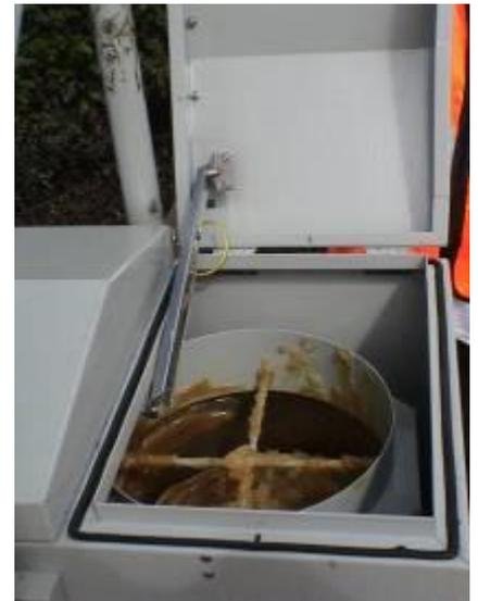
**Note: ensure only approved grease enters the reservoir. Any non-approved materials could severely damage the electric pump.**
